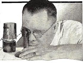
Here is shown the method of using the simple Foucault apparatus for determining the spherical aberrations of the mirror. All that is needed in the way of materials are a light, a can, a piece of tinfoil and an old razor blade. This will give very accurate results.
