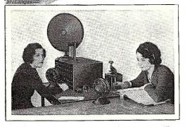
At the stenographic end of the microphone circuit over which letters, contracts, etc., are received from offices. When office door opens a light flashes on the switchboard. If occupant is out the operator takes the message.
