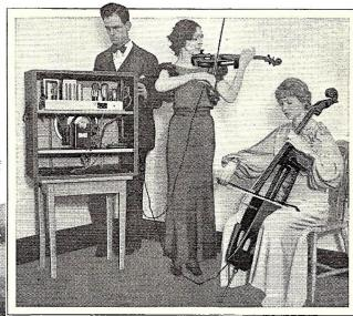
A recital being given with one of the new violins and cellos. Output of the pick-up is here seen utilizing amplifier and speaker of ordinary home radio set for reproduction. Volume from violin fills auditorium.
